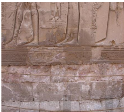
Fig. 3. Field photograph showing salt efflorescence and damage in Luxor temple
